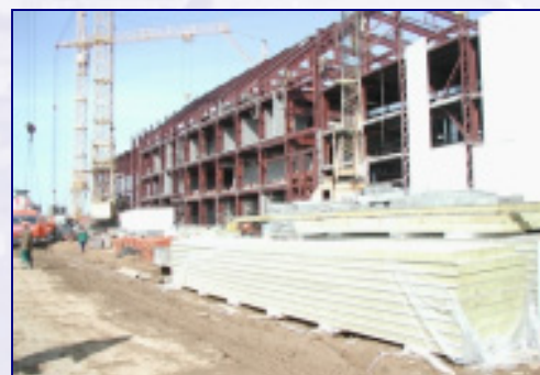
Erection of RTS 'Tereshkovo' (may 2003)
