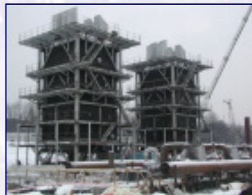
Erection of RTS ‘Tereshkovo’ (february 2003)
